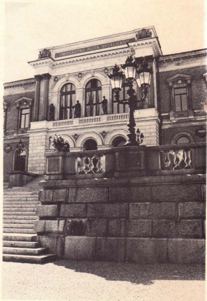
The University Building, Uppsala (Close-up)
