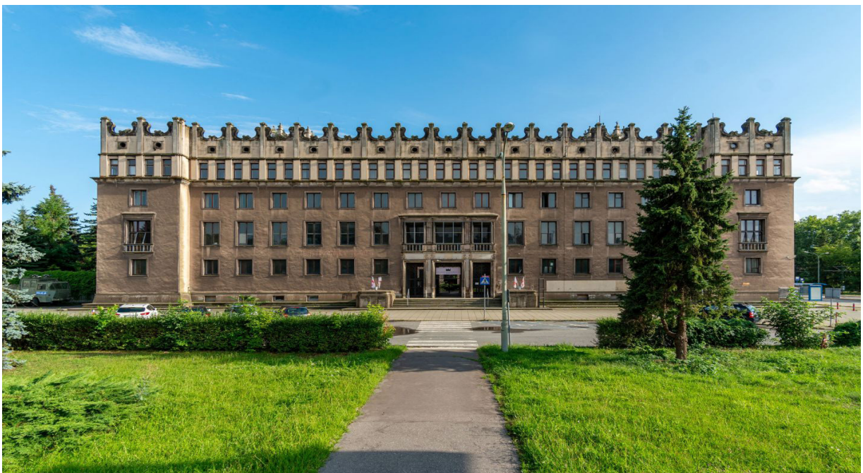
Nowa Huta Administrative Centre (current state). Photo: Jacek Złoczowski
